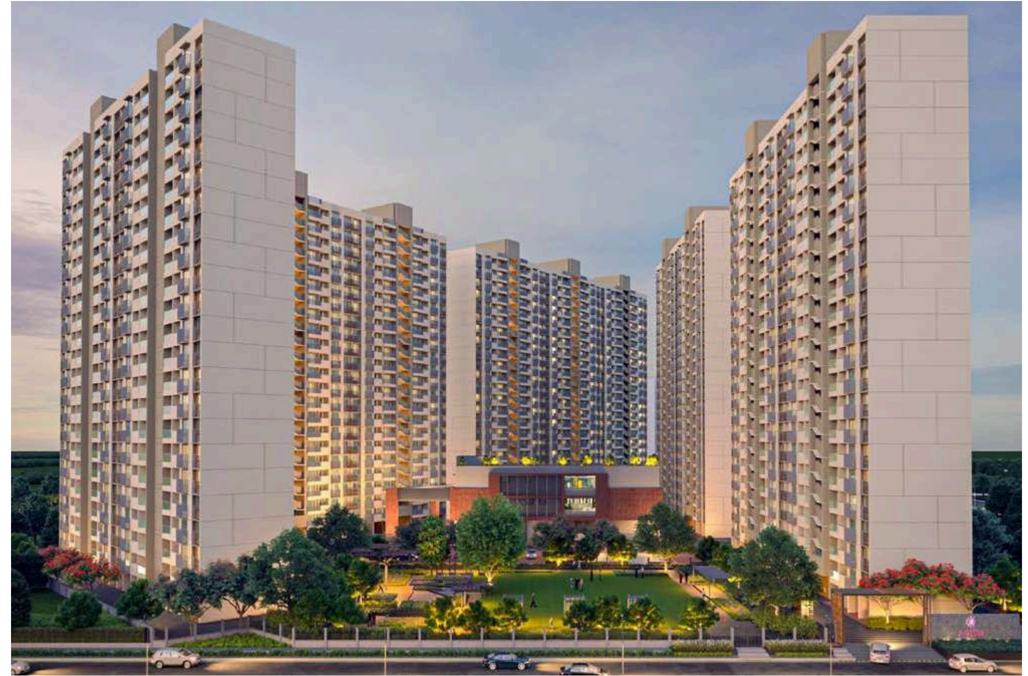
Open Plot adjacent to the Project is P & G Plot and is not a part of the Project. | Artistic Impression
