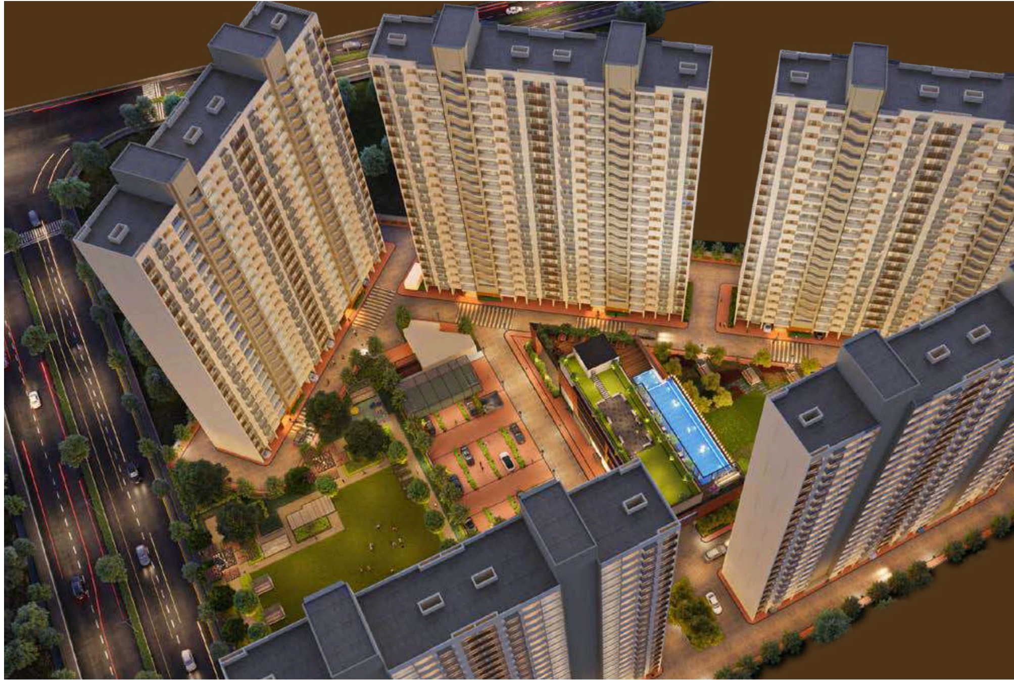
Open Plot adjacent to the Project is P & G Plot and is not a part of the Project. | Artistic Impression
