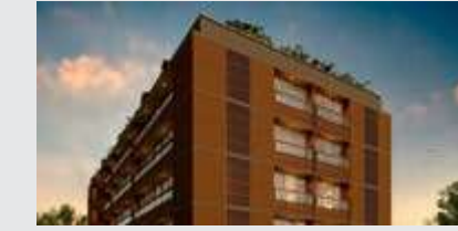
ISHWARMAGNA - 3BHK APARTMENT, MITHAKHALI, AHMEDABAD
